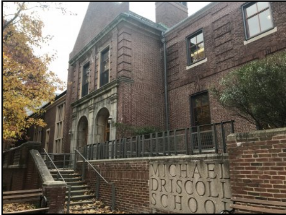
Main entrance to Michael Driscoll School along Westbourne Terrace.
