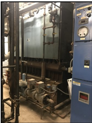
Michael Driscoll School boiler room.
