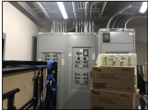
Michael Driscoll School electrical room.
