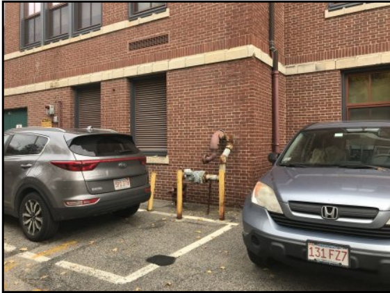
Gas fixtures into the Michael Driscoll School on the southeastern side of the building.
