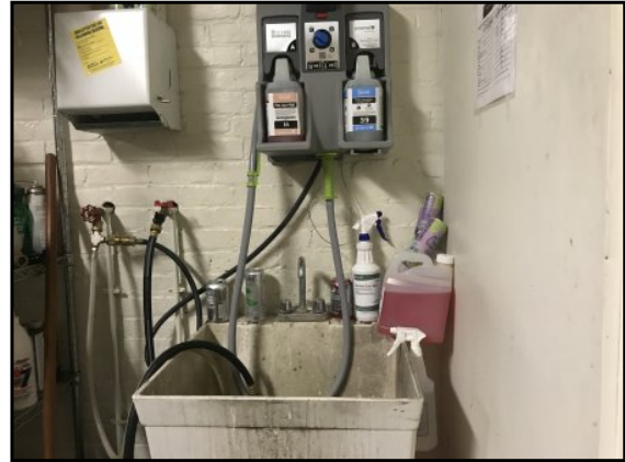
Janitorial wash sink.
