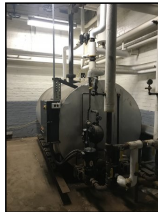
Michael Driscoll School boiler room.
