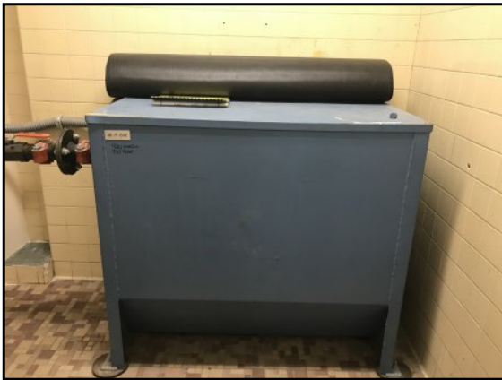
Michael Driscoll School elevator room hydraulic oil tank.
