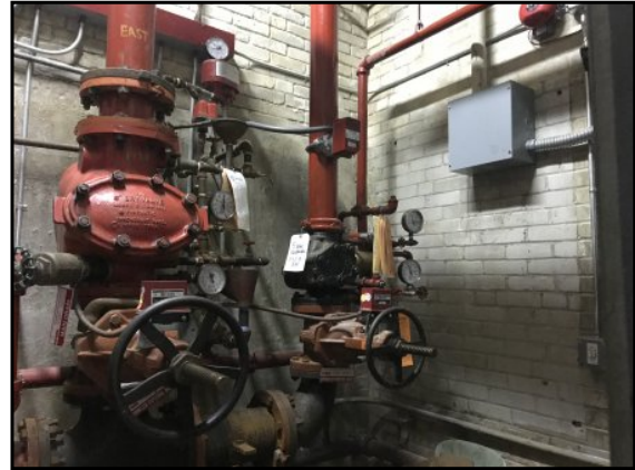
Michael Driscoll School sprinkler system.
