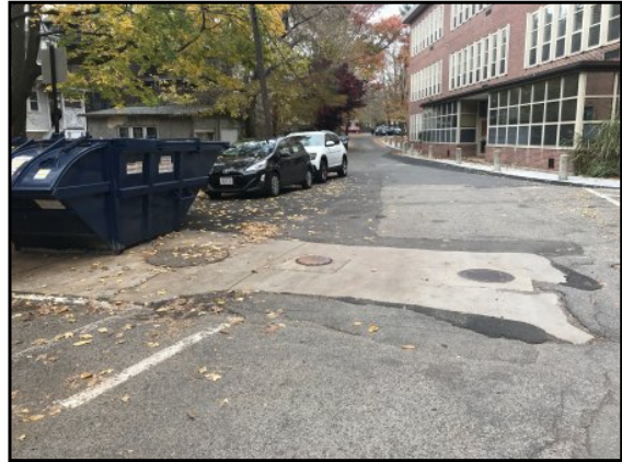
Fill caps for UST located on the southeastern side of the Michael Driscoll School.
