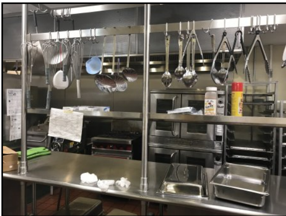
Michael Driscoll School cafeteria kitchen.
