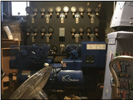
Michael Driscoll School compressor room.
