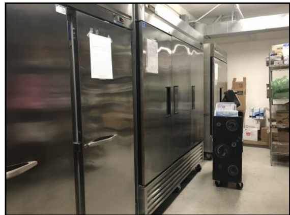
Michael Driscoll School cafeteria freezers.
