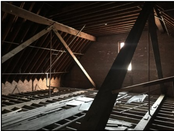
Michael Driscoll School attic.
