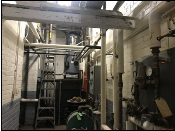
Michael Driscoll School boiler room.
