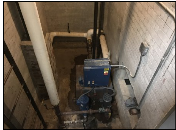
Michael Driscoll School steam compressor.
